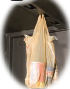
Hooks cut into top support channel inside the locker hold bags for access and organizing supplies.
