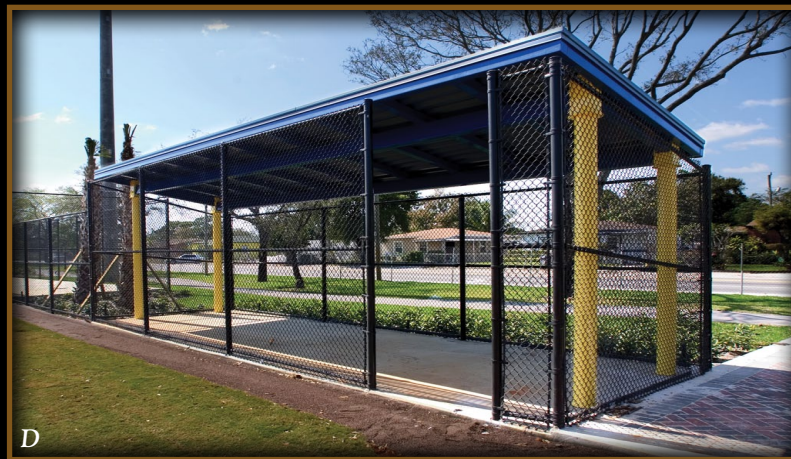
Joseph C. Carter Park, Ft. Lauderdale, FL: 9'-7" x 29' Custom Dugout w/ round columns & standing seam roof.
