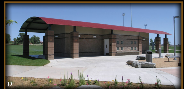
Thornton Community Sports Complex, Thornton, Colorado: 30' x 76' custom Colorado restrooms model with corrugated roof.
