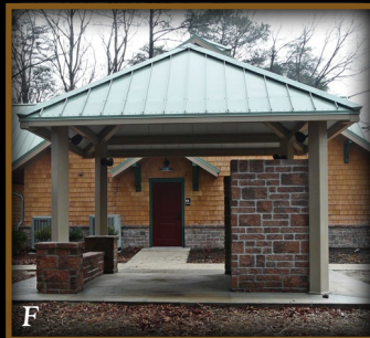
16' x 16' Custom Mesa model concession cover w/ 12" o.c. standing seam steel roof.
