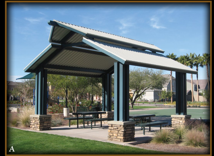
A Homestead Community Park, Phoenix, AZ. 20' x 20' structure with 4 cluster columns and "Parchment" color HR-36 steel roof.
