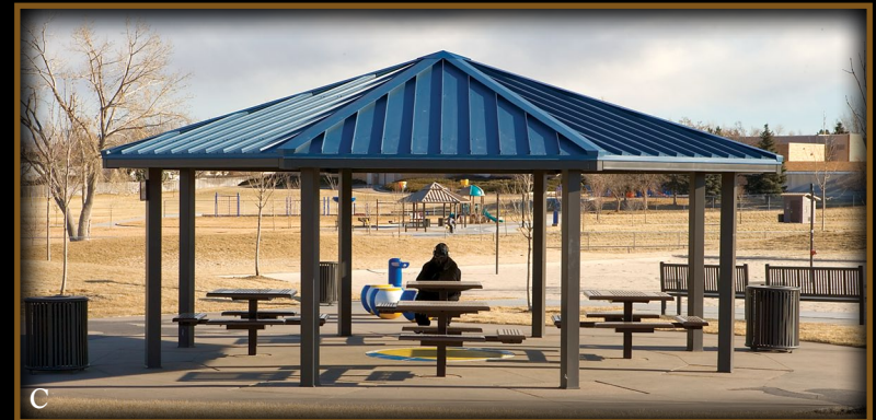
Olympic Park, Aurora, CO: This rugged 24' model features a Regal Blue 12" o.c. standing seam steel roof with tube steel fascia. Two-tier Charleston shown beyond.
