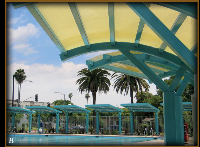
B Pacific Pool, Glendale, CA: 12' x 12' Colorado model shown in foreground with Bright Yellow powdercoated, perforated screen roofing. See background Marana/Solar structures on page 64.
