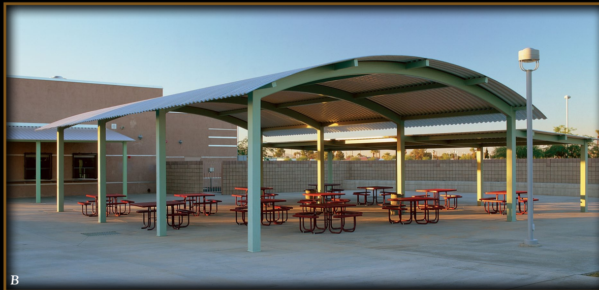
East Valley Academy, Chandler, AZ: This 36' x 51' high school lunch pavilion has a curved roof of 24 gauge HR-36 galvalume steel with no trim, with attached 15' 6" x 51' Sierra model. The shelter design complements the art deco campus architecture.
