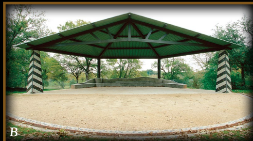
B Community Park, Austin, TX: This 45' model features R-panel roof with tile mosaic columns by Twyla Arthur.
