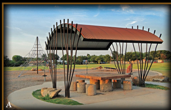
A LBJ Park, Grand Prairie, TX: 15' x 15' Ocotillo model with corrugated steel roof in Copper Penny color..
