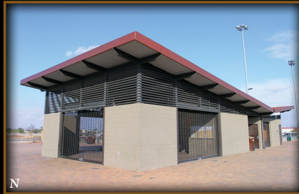
Festival Fields, Avondale, AZ: 40' x 82'-8" Custom restroom & concession w/ block walls by others. (Water harvesting roof)
