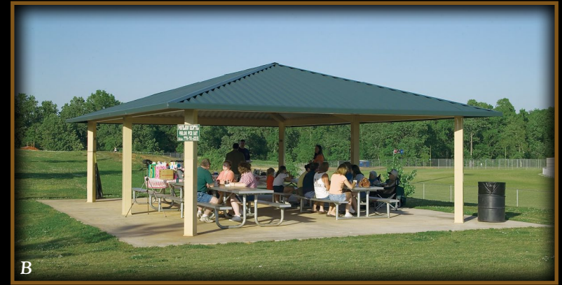
B Community Sports Park, Cummings, GA: This economical design stands up to heavy use and keeps looking great. 24' x 40' model shown with Forest Green HR-36 steel roof.
