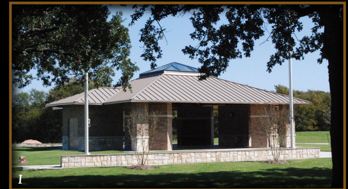
Rolling Oaks Memorial Center, Coppell, TX: 47'-10" x 61'-5" Custom Mesa pavilion w/ cedar T&G sub-roof under standing seam steel roof.
