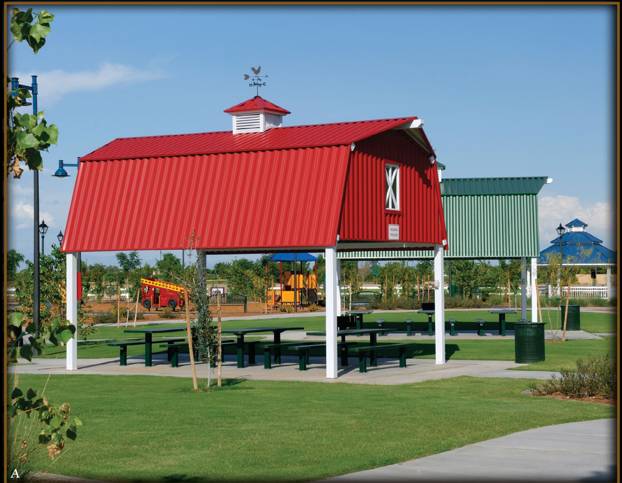
Tumbleweed Park, Chandler, AZ: 16' x 21' Heartland models with 24 ga HR-36 steel roofs in Bright Red & Evergreen colors with cupola's and provision for weathervanes. (20' Dallas model in background to right)
